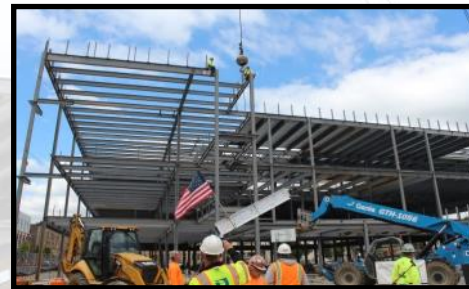
Passaic Leonard Place Elementary School Beam Signing
