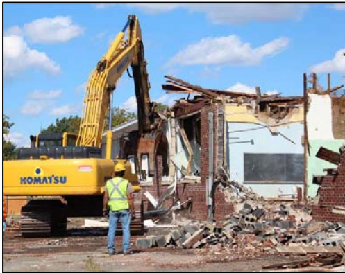
Demolition Activities at Caruso Elementary School in Keansburg
