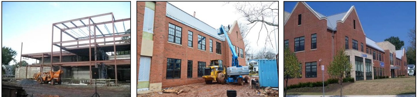
Construction of Victor Mravlag Elementary School
